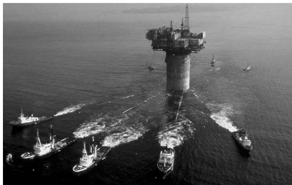
FIGURE 9 Boats tow a concrete platform to a site in the North Sea.
